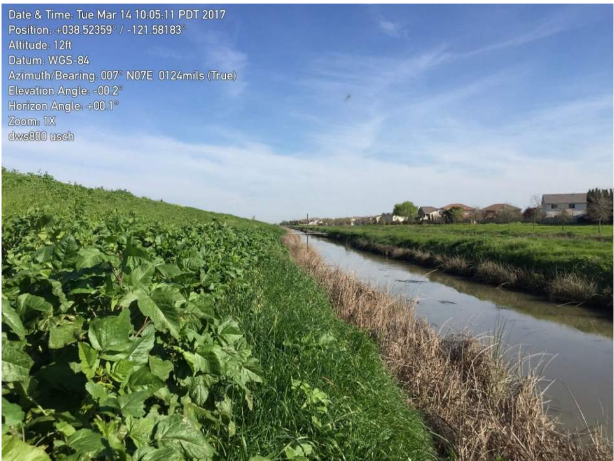
Photo 10-11. Toe Drain – Typical Conditions
